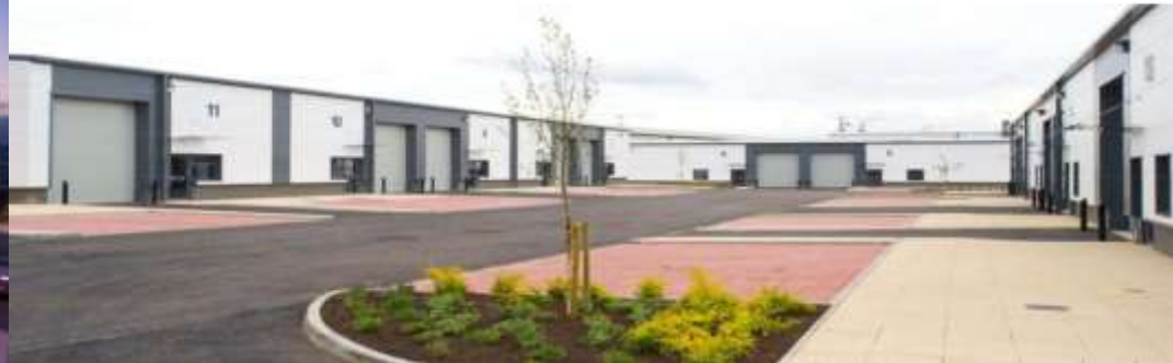
West Chirton Industrial Estate, North Shields
